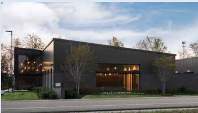
Elevated design industrial use that addresses the primary street.
