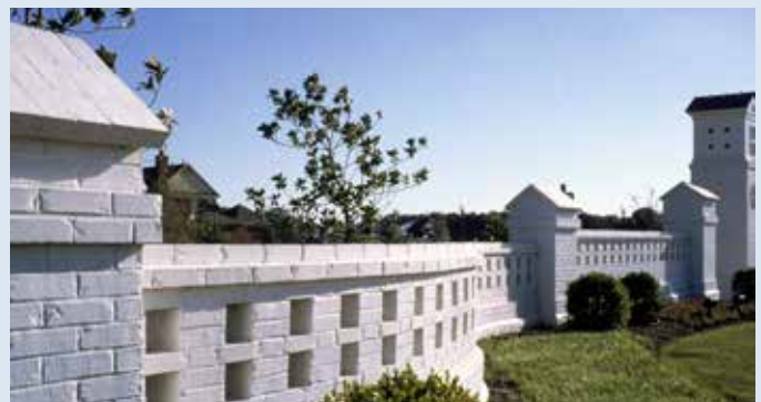
Emphasis at a development entry from the Gateway Corridor
