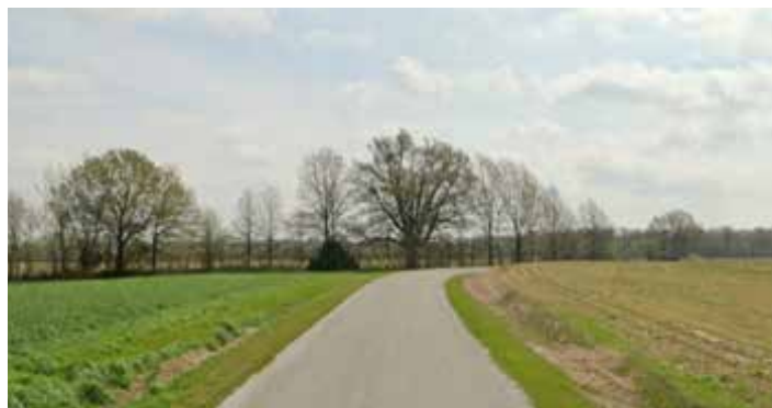
90-degree curve and lack of shoulders on Elm Tree Road
