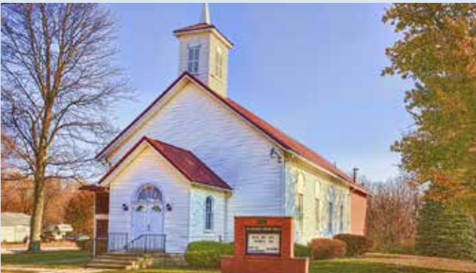
Churches and other civic/institutional uses should address the primary street and provide parking to the side or rear.
