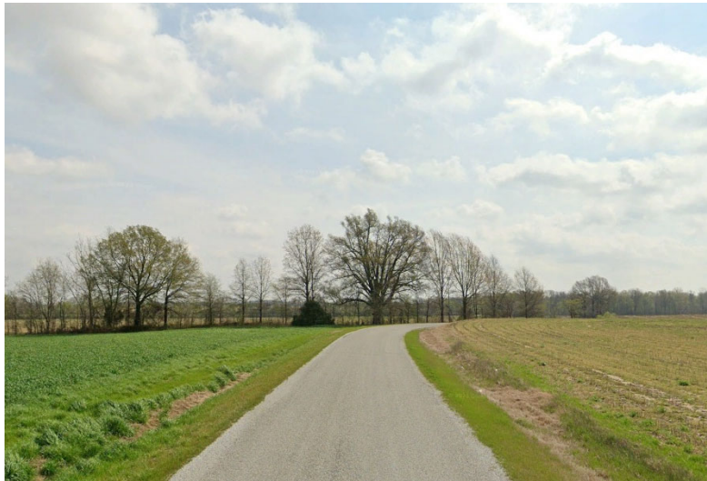
90-degree curve and lack of shoulders on Elm Tree Road
