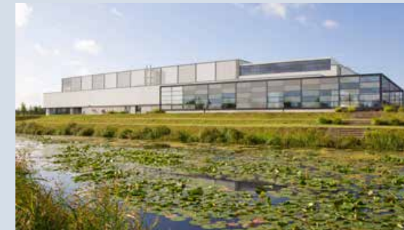
Industrial Site with Stormwater Feature
