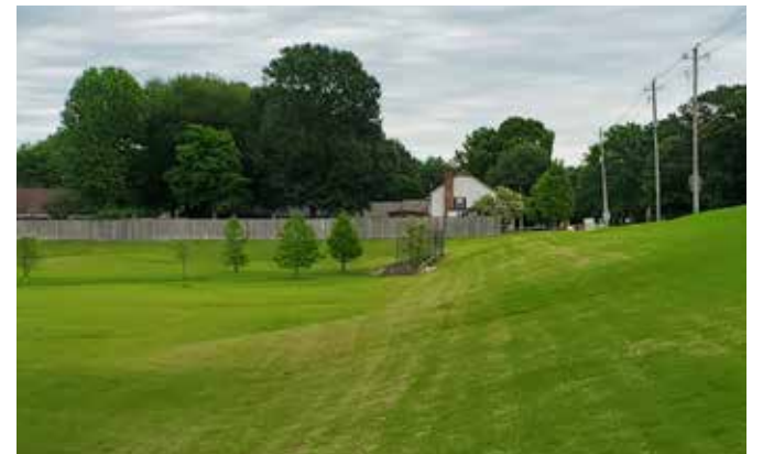
The design and landscape of the stormwater pond in this image was not implemented in a way that enables it to serve as a more natural feature or amenity.
