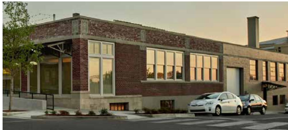
Breweries and distilleries often incorporate public gathering spaces both interior and exterior and may be accompanied by large-scale equipment located adjacent to the building. Proper screening and placement of such elements can restrict sightlines to equipment.
