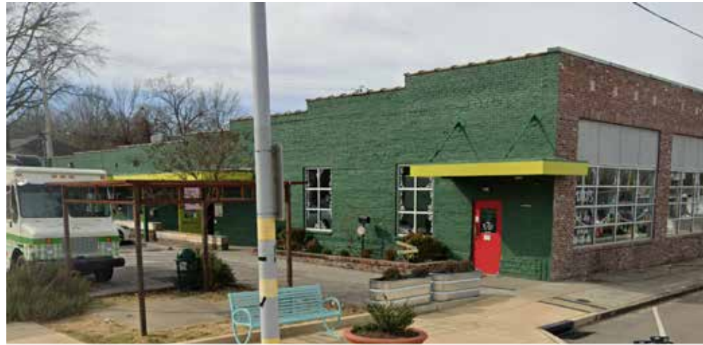
Redevelopment of an existing building with storefront that addresses the primary road and provides adjacent open space for customer pick-up and gathering for events.
