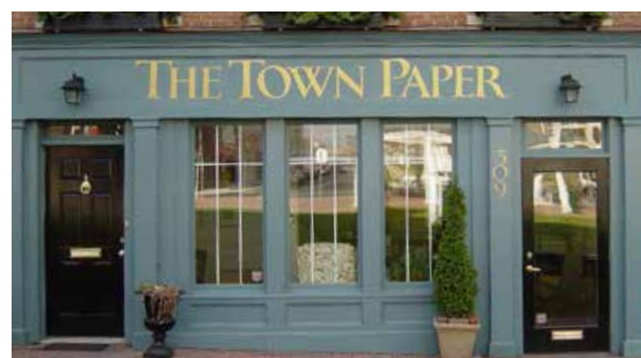
Storefront entrance is clearly distinguished from those serving the floors above.
