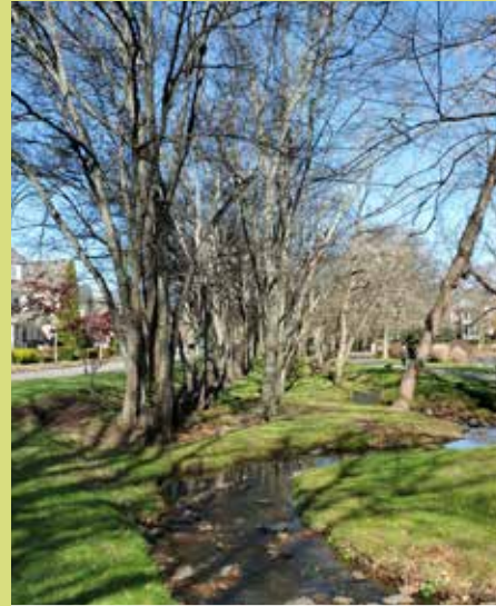
A more 'natural' approach to stormwater management.
