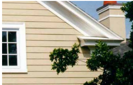
Classic cornice and rake detailing with cornice returns provide a timeless quality to this gable form.
