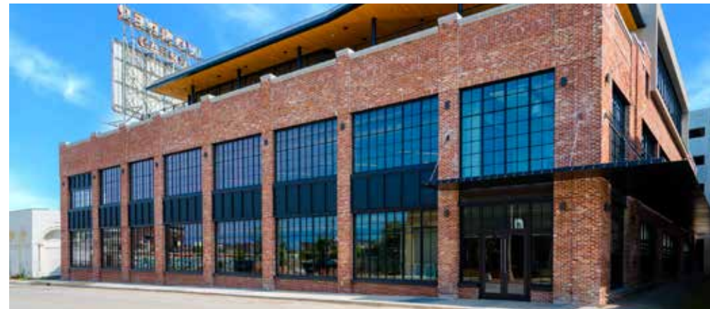
Office building incorporates a simple rhythm of bays and recesses to break up a lengthy facade. Canopy enhances primary entrance; appropriate ground and upper floor transparency.
