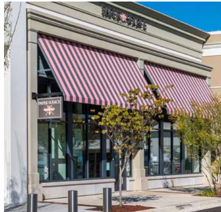
Bollards, street trees and a high degree of ground floor transparency result in a comfortable and engaging space.
