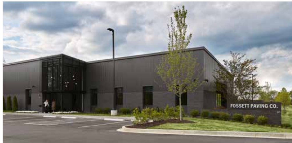
This industrial building features a clearly defined entrance which also serves to break the mass, materials that emphasize both hierarchy and base while providing human scale, vertical orientation of windows and appropriate monument signage and landscaping.
