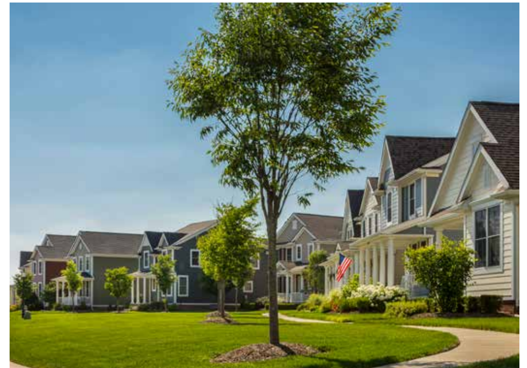
Homes should front on neighborhood greens, parks and amenity spaces thus strengthening the sense of community and providing passive safety through "eyes on the street".
