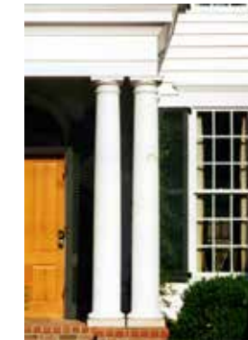
An example of an appropriate well detailed column capital, frieze, and cornice.
