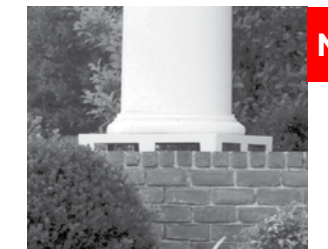
Visible aluminum vent blocks are inappropriate.
