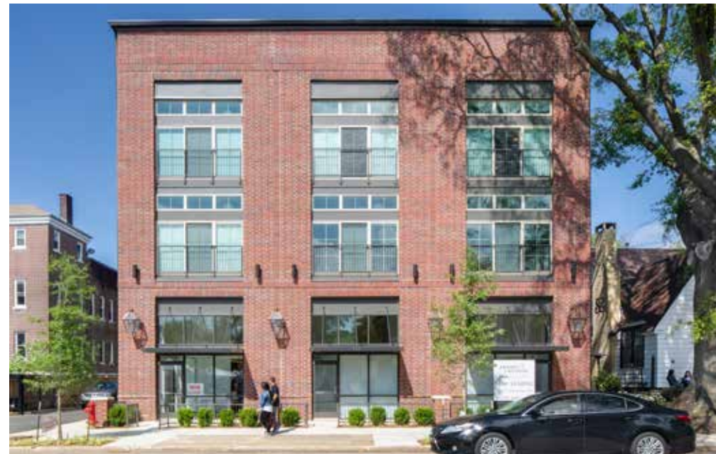
The mixed-use building in this image addresses the street in a way befitting a Town Center. Appropriate design elements include storefront design for ground floor live/work space, appropriate streetscape including street trees, and a clean use of material and three-part hierarchy.
