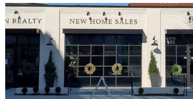
Consideration will be given to alternative storefront designs including the use of folding or sliding doors.
