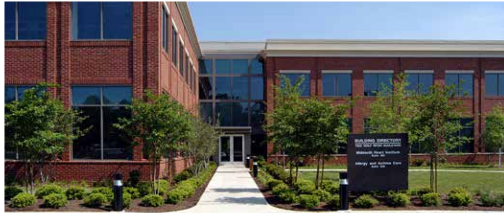
The building engages the front sidewalk, incorporates good transparency, a clearly defined primary entrance, and well proportioned signage and pedestrian scale lighting.
