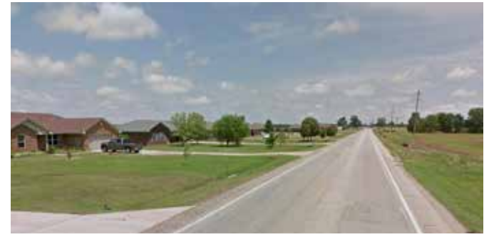
The image above depicts homes lining a road in a way that does little to enhance or preserve the surrounding rural character. This image was the least preferred for countryside roads in the Community Vision Survey.
