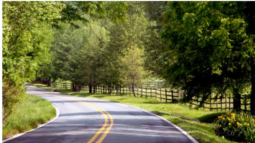
The image above incorporates several features of an Enhanced Scenic Buffer Zone along a rural roadway including preservation of specimen trees, a 3-rail fence, and graded swale that also serves as a shoulder.
