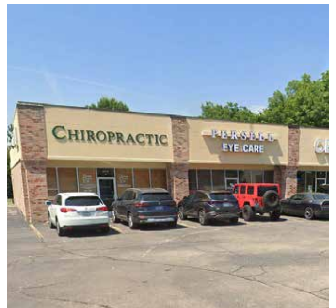
This strip center lacks architectural character, a defined pedestrian realm, and landscaping. This image was the least preferred for Four-Ways in the Community Vision Survey.
